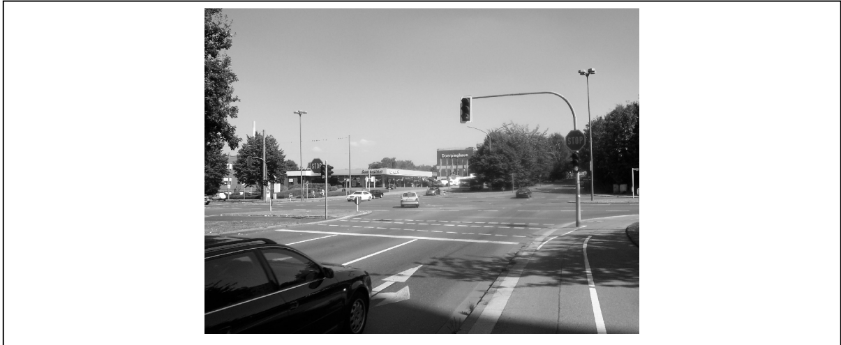
Fig. 4: Problem area for older drivers: Huge signalled intersection with left-turn and simultaneously oncoming straight traffic
