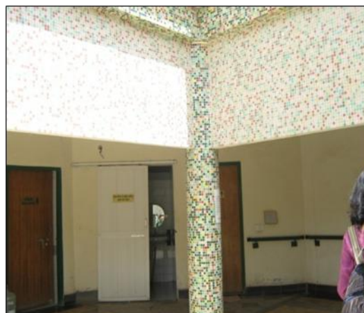
Figure 2: Contrasting colors are used for wall finishing, this help people with visual impairments in identification of spaces.
