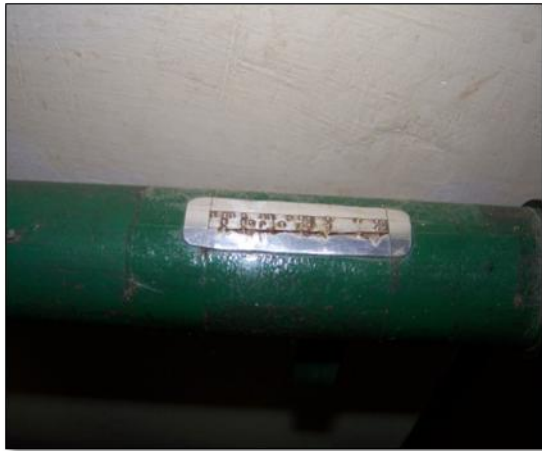
Figure 1: The guide rail is provided with Braille script. This guides visually impaired to walk throughout the campus.
