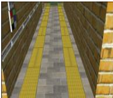
Fig 6.2: tactile tiles as the flooring material
