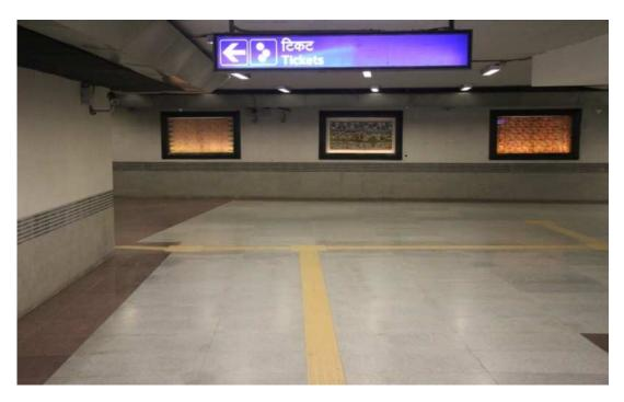
Photo 3 Tactile tiles for guiding the vision impaired at a Delhi Metro Rail Station
