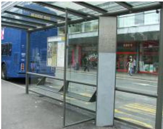
Fig 14 Glass bus shelter with no contrast bands
