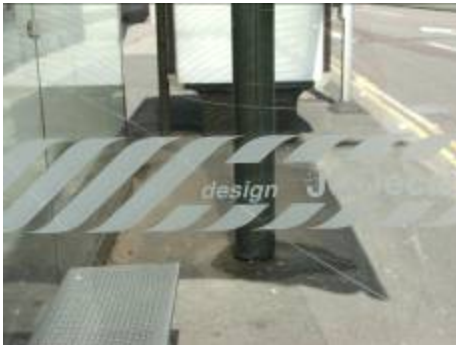
Fig 34 Details of undetectable glazed manifestations
