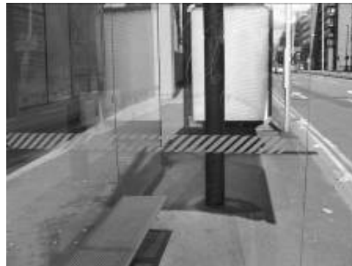
Fig 25 No protection edge on the glass panels
