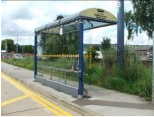
Fig 20 Bus shelter with a protection band at the bottom
