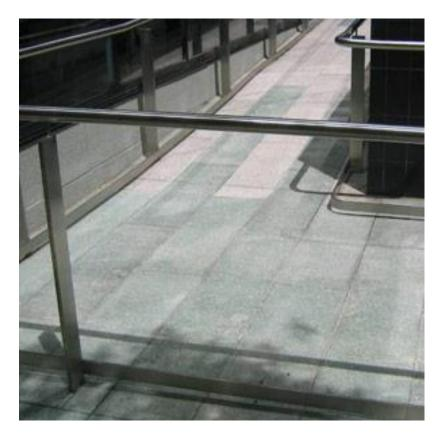
A ramp with appropriate handrails and kerb rails Image via Australian Human Rights Commission; links to source
