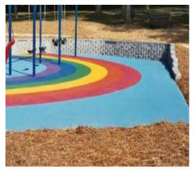
Photo 4. Unitary Synthetic Materials can add interest to the playground's surfacing with colors and shapes. Photo courtesy of Boundless Playgrounds.
