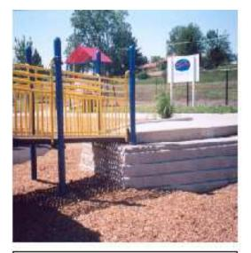
Photo 5. A smooth transition from an accessible surface to the entrance is needed for fully integrated play. Photo courtesy of Boundless Playaprounds.
