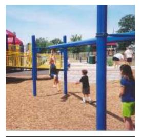
Photo 3. Loose materials move on impact and provide protection for the most severe playground injuries. Photo courtesy of Boundless Playgrounds
