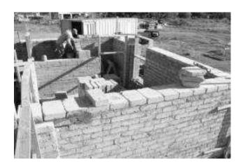
LMI-1 Prototype, Series 012 Universal Home™ design- Abilene, Texas. First HUD funded Lime stabilized Compressed Earth Block Home in US History. Constructed in 2010. COURTESY PHOTO
