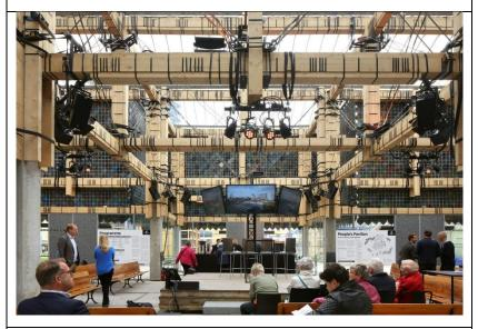
People's Pavilion at Dutch Design Week - made with borrowed timber and designed for recovery of materials
