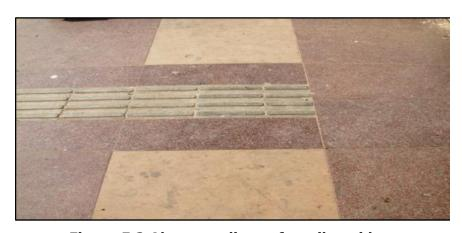
Figure 5.2 Abrupt endings of tactile guide ways
